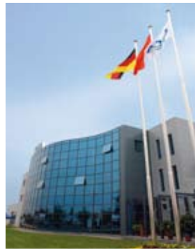
GEA Power Cooling Technologies Langfang, China
