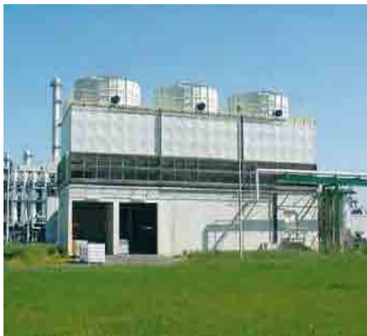
CMDI cooling tower type 840 Chemical industrial plant in Belgium
